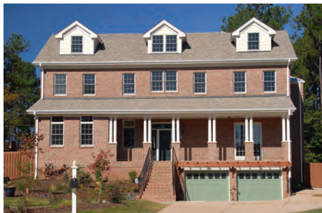
With the use of locally sourced and produced brick, the National Homebuilder Mainstream Green Home was the first LEED Platinum home in the southeast. © Chris Beck
